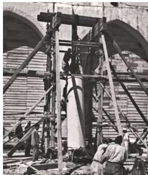
130 Placing a new column IAA 22.011
