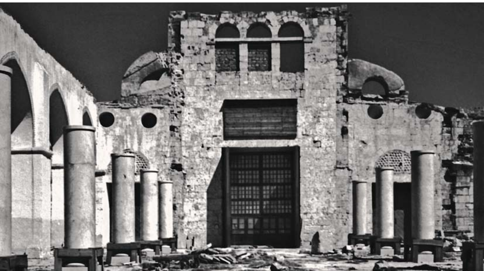
131 Two rows of new columns set up in the nave, near the temporarily freestanding inner northern façade. The monolithic marble columns were imported from Italy. IAA 22.124
