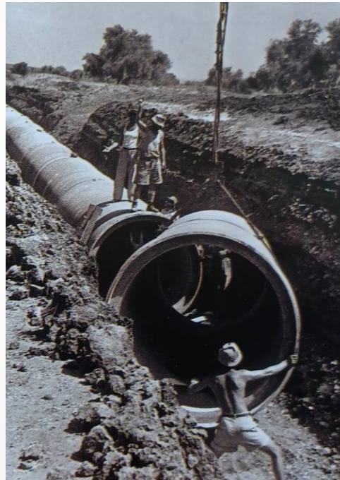
1954 The Laying of a pipe as part of the National Water Carrier
